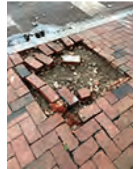
Loose bricks like these are not only unsightly, but a tripping hazard. If you have these, remove and store them or have a mason or arborist secure them in place.
